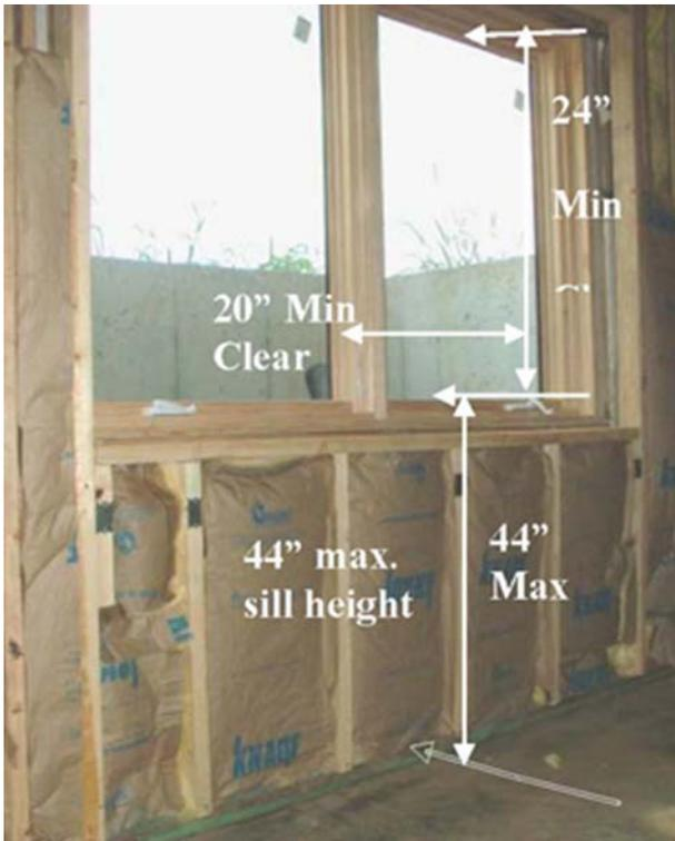
**Emergency escape windows** shall be operational from the inside of the room without the use of keys, tools, or special knowledge. The opening shall have a minimum height of 24 inches and minimum width of 20 inches with the bottom of the openable portion being not more than 44 inches above the floor
