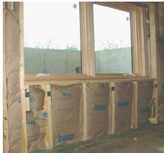
**Windows** – Windows contribute significantly to energy efficiency. New windows shall have an energy efficiency (U-value) of U = 0.35 or less (minimum double glazed window). Single pane windows with storms are not permitted.
