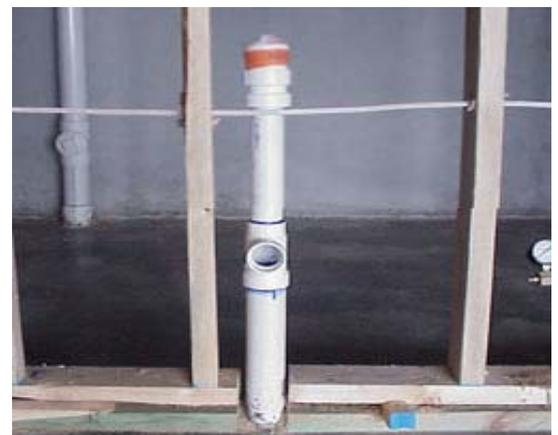
installed at least 6 inches above the flood level rim of the highest fixture being vented.
