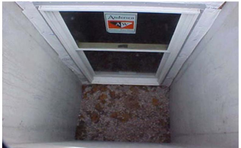
maximum of 6 inches into the required dimensions of the window well. Ladders shall have an inside width of at least 12 inches, shall project at least 3 inches from the wall, and ladder rungs shall be spaced not more than 18 inches on center vertically for the full height of the window well if a cover is provided over the well it shall be openable from the egress side and provide the same clear areas as required for the window.
