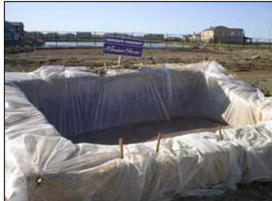
Self-installed washout container w/ 10-mil min. plastic.
