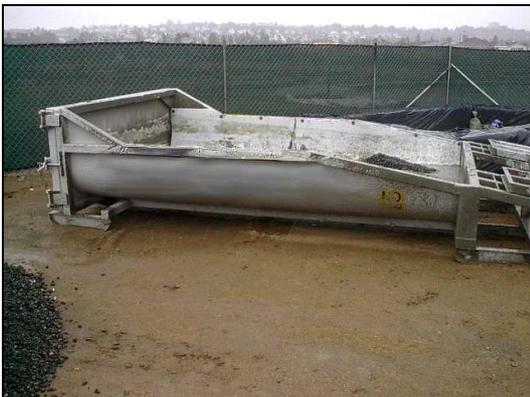
Prefabricated – reusable washout structure.
